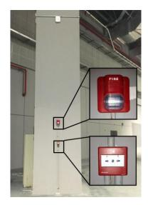
An example of a pillar with manual fire alarm activation button and beacon light with fire siren.
